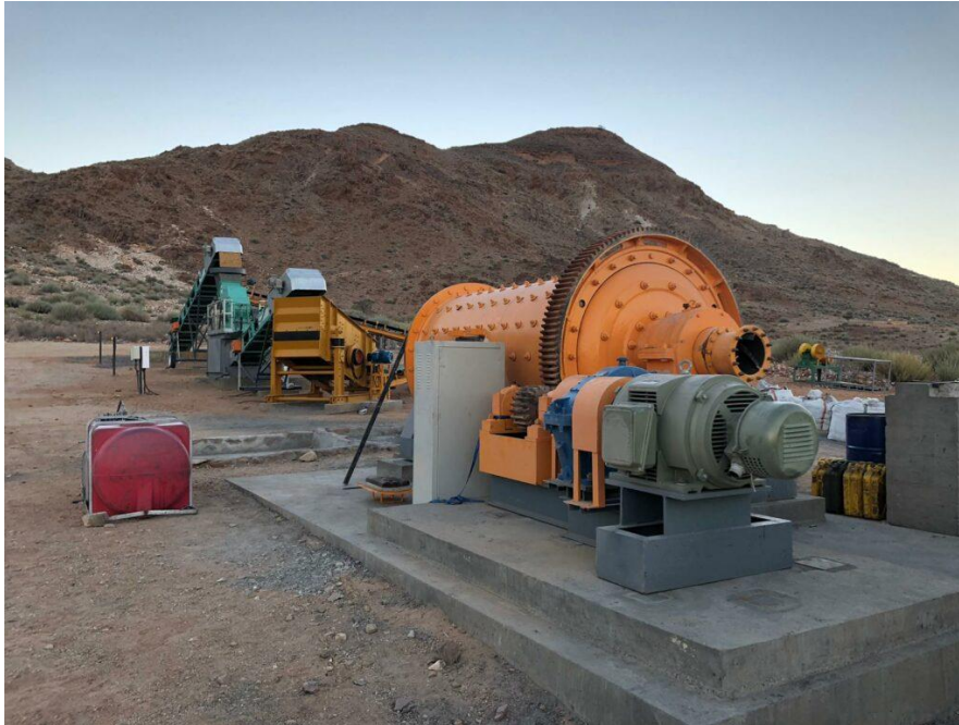
Aukam Plant commercial scale rod mill, screeners and conveyance systems
